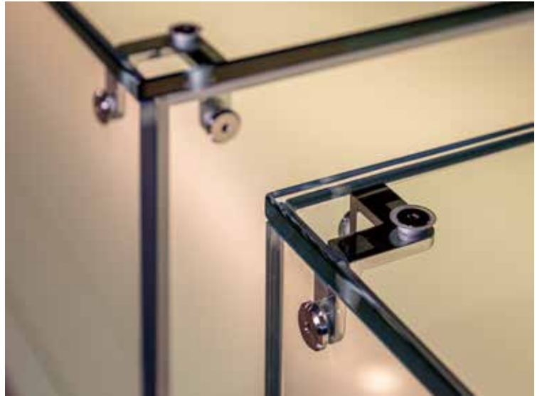
Glass gantry with mechanical clamping
